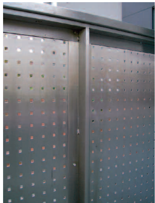
Localized rust staining was caused by iron particles from a disc, which had previously been used on carbon steel (left). If ferrous contamination has occurred, it can be removed by on-site pickling (right) [12]
