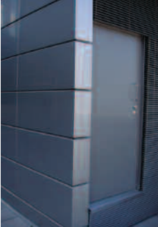
The stiffening effect of the edges ensures optical flatness
