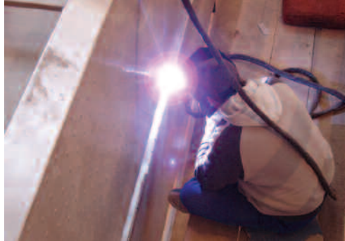
On-site welding of a stainless steel swimming pool structure
