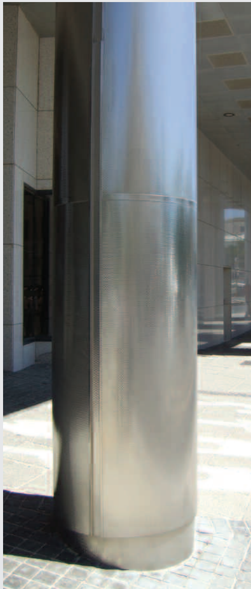
Patterned stainless steel ensures even surfaces and efficiently masks dents
